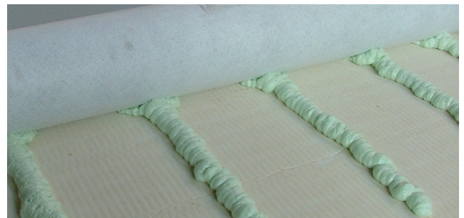
A bonded membrane incorporating HardRock Multi-Fix (DD)
